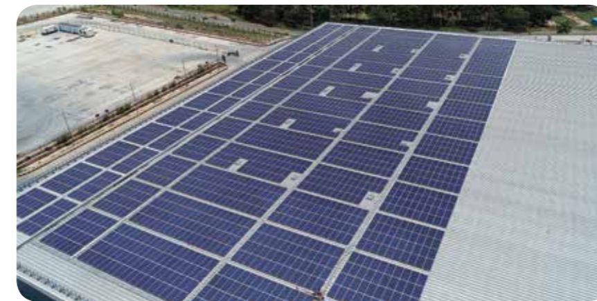
Solar panel installation at the Mysuru Factory
