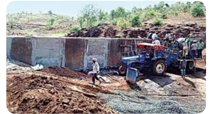
Restoration of the Rojghat check dam
