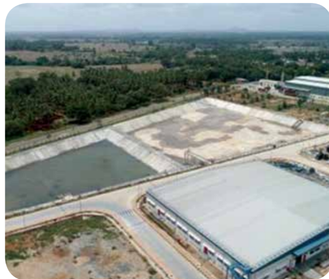
Mysuru factory - Rooftop rainwater collection reservoir
