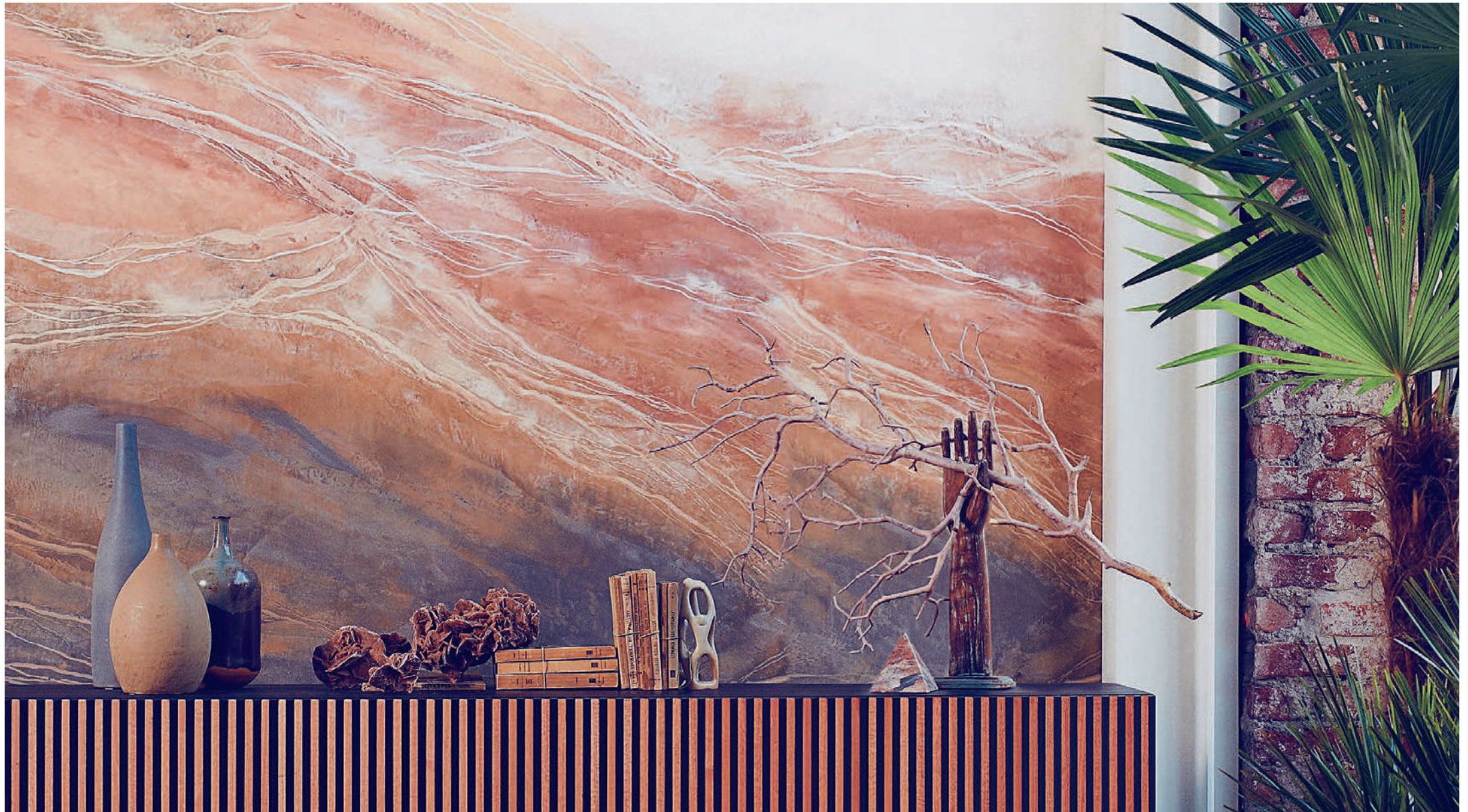
Base Coat - Marmorino White 0908 | Top Coat 1 - Marmorino Copper Coast 8615 | Top Coat 2 - Marmorino Dark Shadow 8294 Top Coat 3 - Marmorino Indian Spice 8568 | Top Coat 4 - Marmorino White 0908
