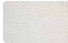
New and existing plasters
